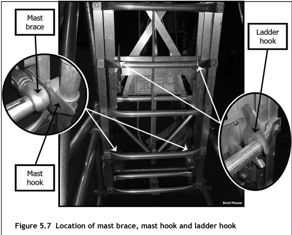
Figure 5.7 Location of mast brace, mast hook and ladder hook
